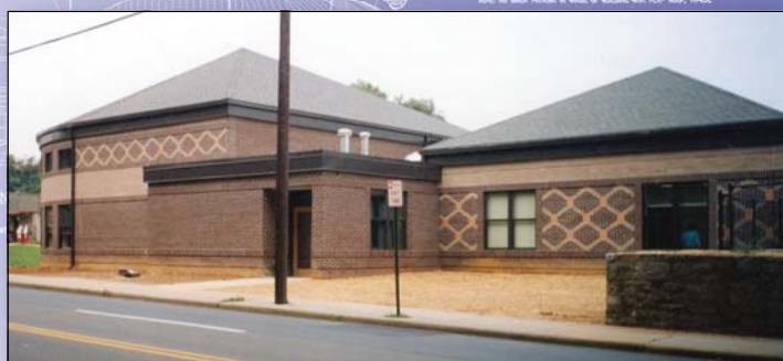
The old house served the community until it was torn down in June 1993 to make way for the current building. Thus began a new opportunity for the JCC to become a cohesive agency ready to take on the challenges of the future - serving not only the Jewish community, but the greater Asheville community.
