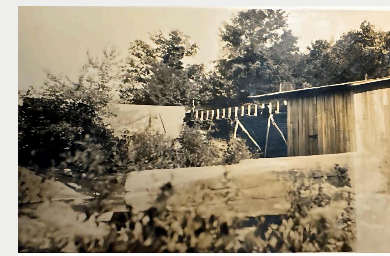
Dam and Battery Building
