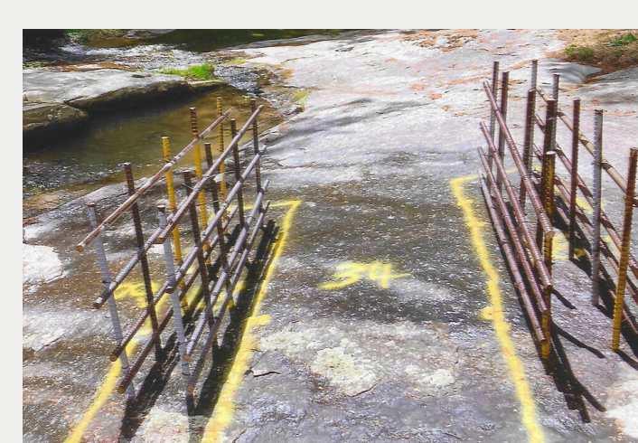
New Water Wheel Supports
