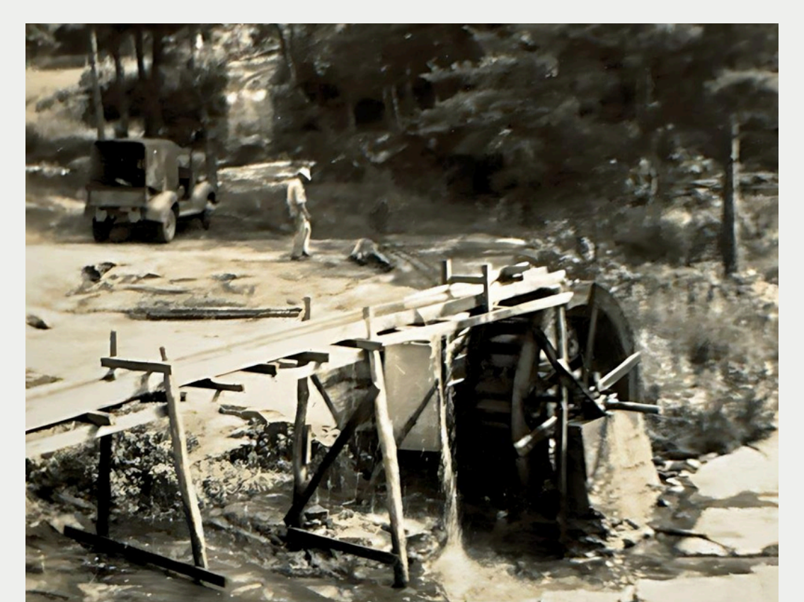
Ambrose Dismantling Power Plant
